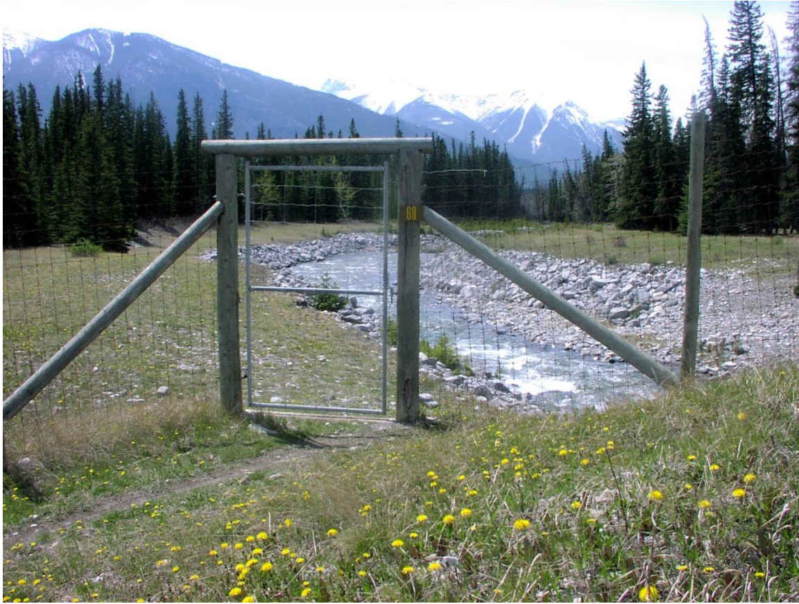
Single swing gate in wildlife exclusion fence (Photo: Tony Clevenger).
