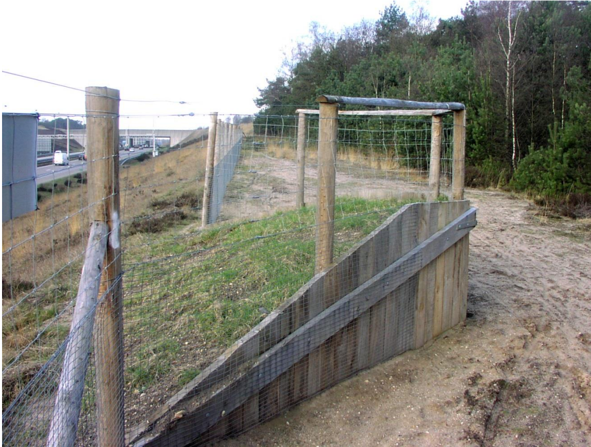
Wildlife "jump-out" escape ramp (Photo: Tony Clevenger).
