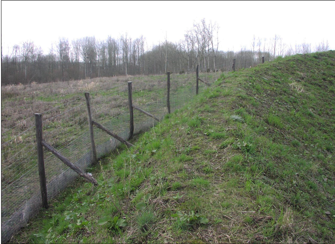
Berm on wildlife overpass (Photo: Tony Clevenger).
