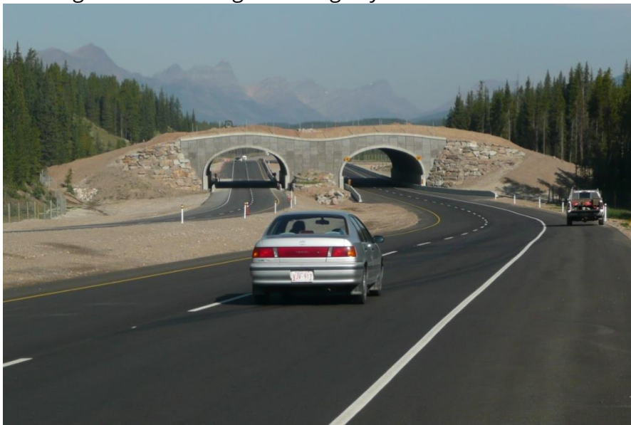
Recently completed wildlife overpass without landscaping (Photo: Tony Clevenger).
