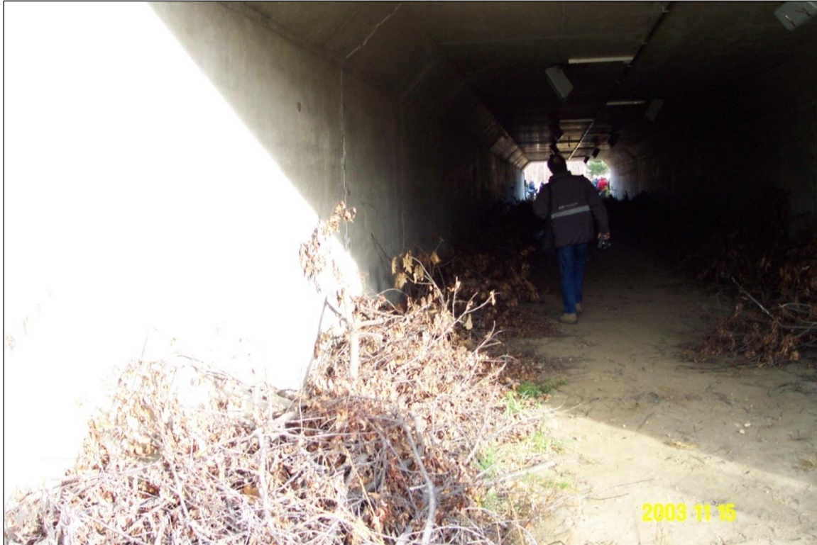
Brush and root wads placed along underpass wall to provide cover for mammals (Photo: Nancy Newhouse).
