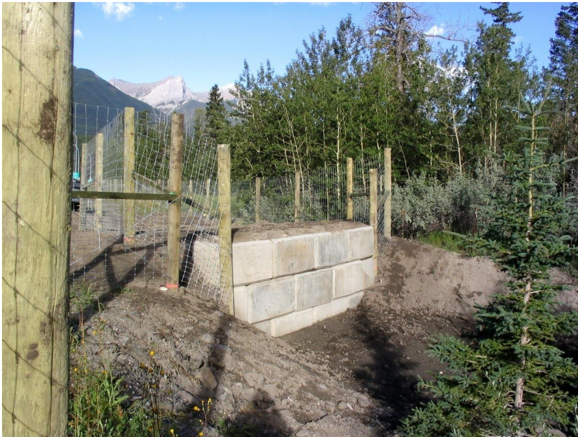
Escape ramp (jump-out) for wildlife trapped inside highway right-of-way (Photo: Tony Clevenger).
