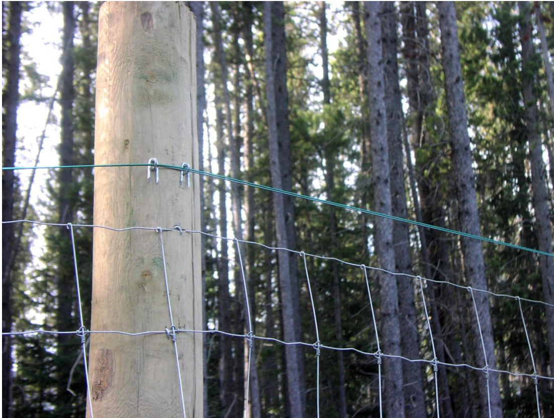
High tensile cable designed to break fall of trees onto fence material (Photo: Tony Clevenger).
