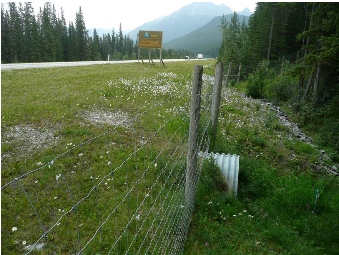
Wildlife exclusion fencing and culvert design wildlife underpass (Photo: Tony Clevenger).
